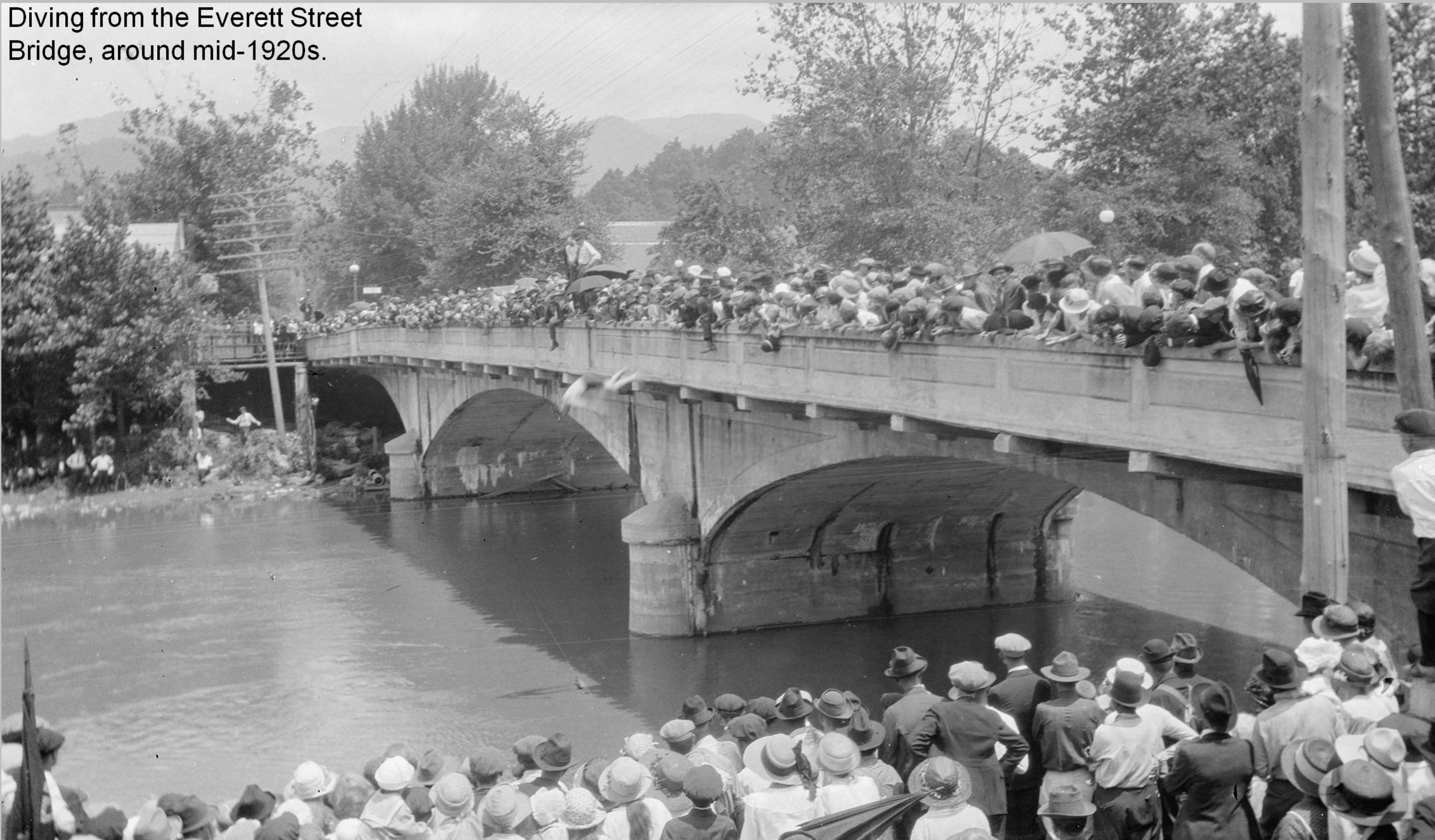
Quite a crowd had gathered on and around the Everett Street Bridge, apparently to watch diving (note the blurred image just to the left of the concrete support). A multitude of telephone wires, with one bare uninsulated wire per phone line, pass overhead and loop around insulators on the six beams affixed to the pole on the north side, next to the Sim DeHart store.
